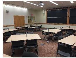
Pettengill G65 New Flip-top Rolling Tables Ductwork changes to Reduce Air Noise
