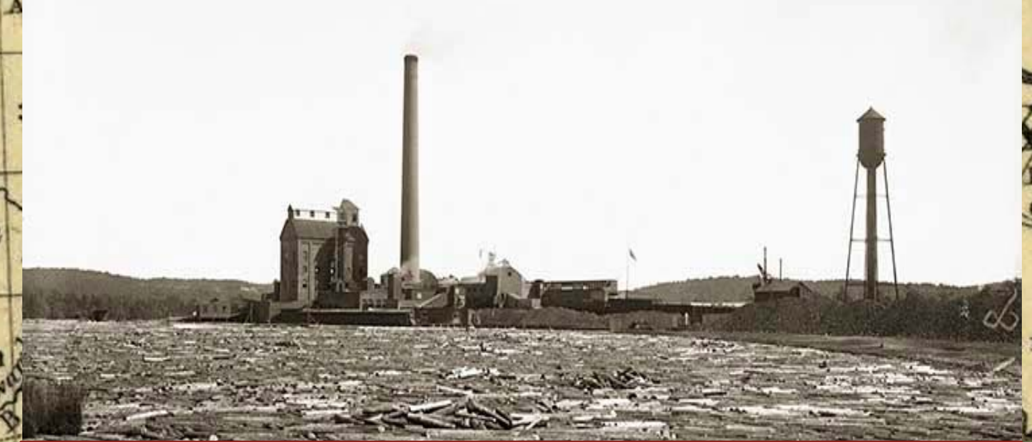
Log jam on the St. Croix preventing travel between Pleasant Point and Indian Township
