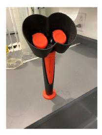
For the eyewash station on the left, pull the lever on the left to activate the water. For the eyewash station on the right, push the red vertical button. For either type:
