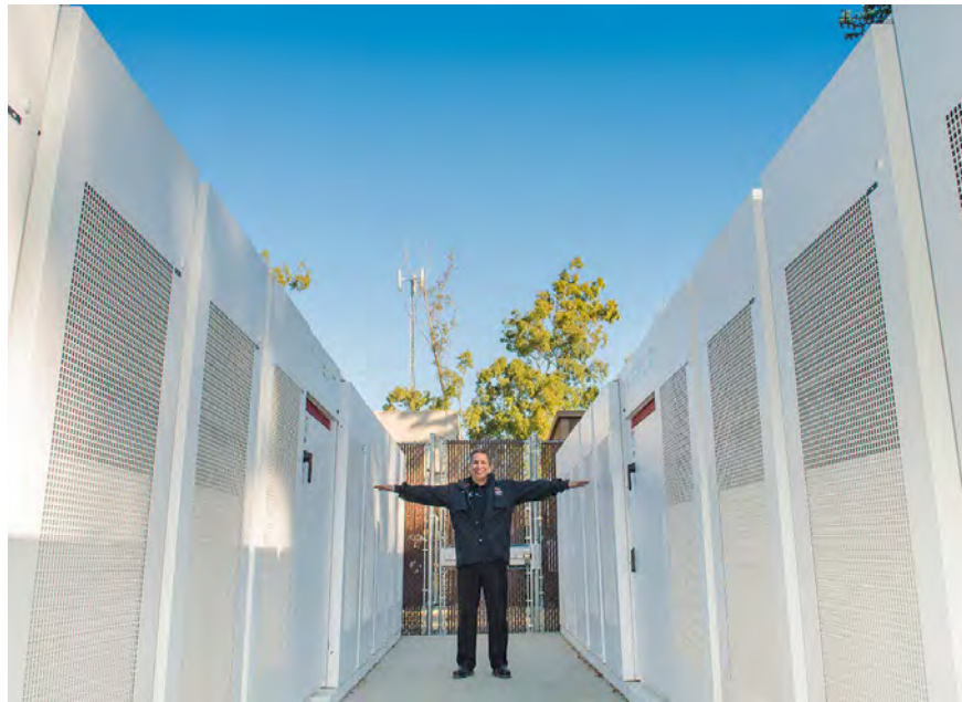
Kenny Seeton, central plant/energy manager at CSUDH, stands among 20 Tesla battery banks. Photo credit: CSUDH Office of Communications
